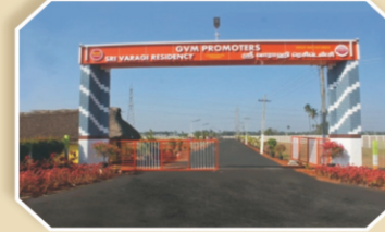
GRAND ENTRANCE GATE WITH ARCH
